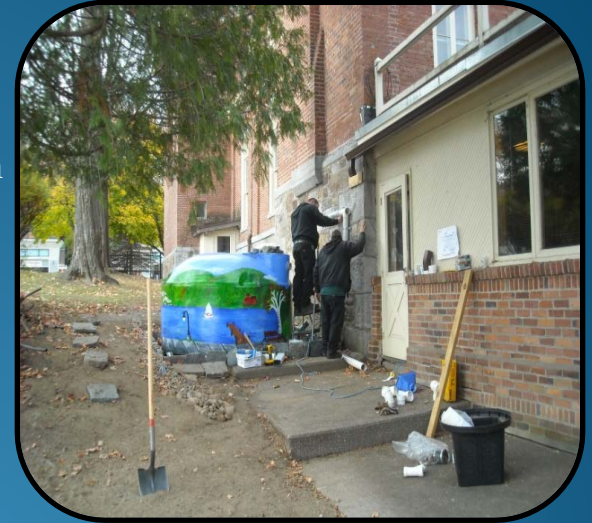
Attachment of collection pvc conduit "bridge"
