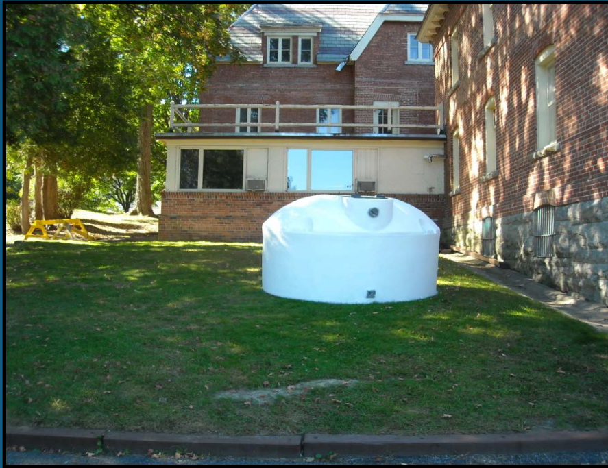
Arrival and prep of the roof water collection cistern (1,100 gal) with Town of Lake George Buildings and Grounds Personnel
