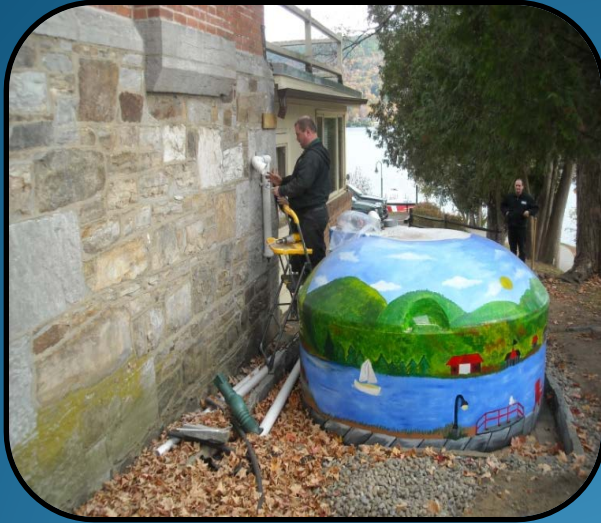
Attachment of collection pvc conduit "bridge"
