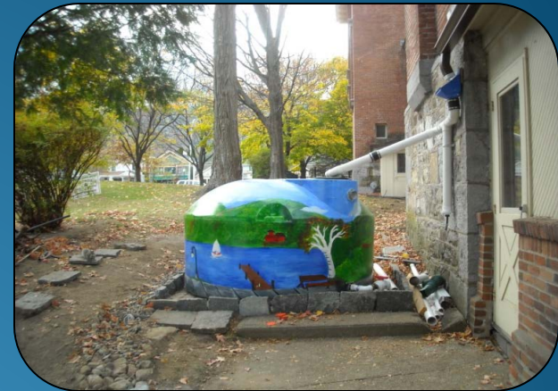
Connecting roof gutter with cistern
