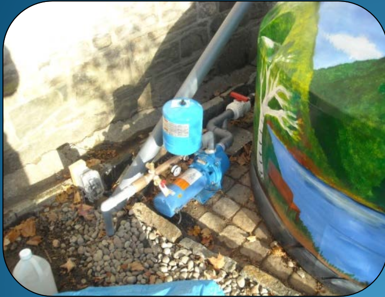
Pump Assembly Installed. 1.5 horsepower inline pump
