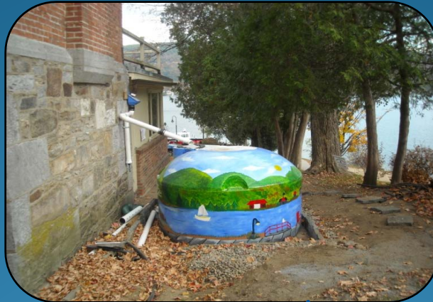
Connecting roof gutter with cistern
