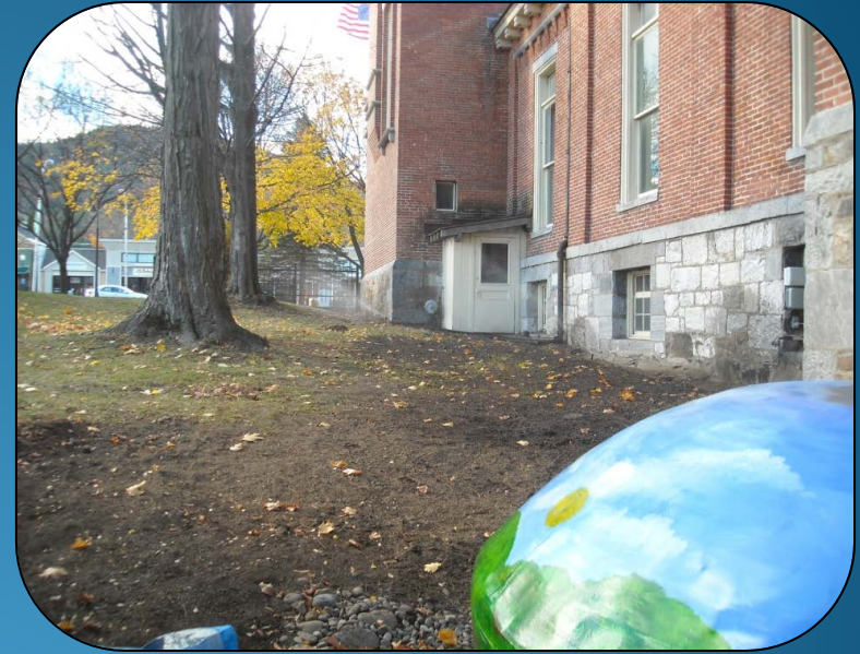
Irrigation Zone #3 installed and functioning
